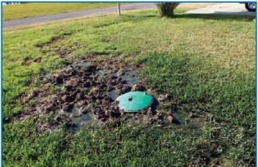
Figure 3: Surfacing of untreated wastewater around a failing OSSF.
